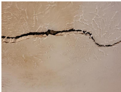
1635-3 Drywall/Joint Compound Interior Walls/Ceilings
